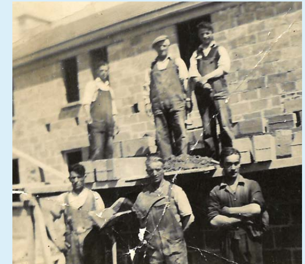
Building local authority housing in Dundalk, 1950 ( Louth County Archives )
