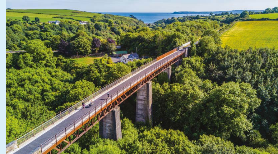
Ballyvoile Viaduct on the Waterford Greenway, (Waterford City and County Archives)
