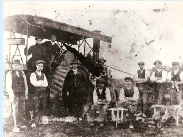
Road workers at Ballygar, Co. Galway, c. 1940 (Galway County Council Archives)
